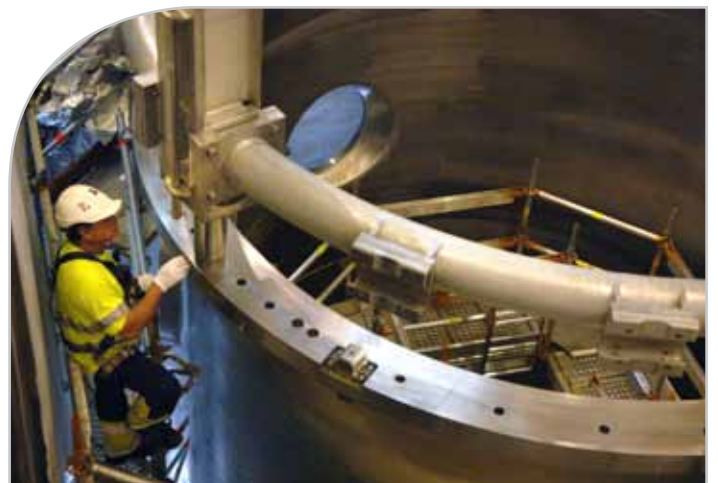
Lower Internal Introduction in the RPV
