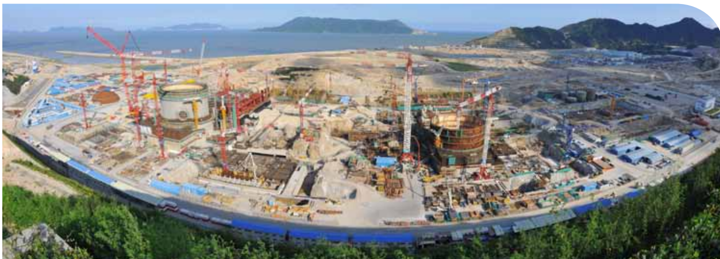
General View of Taishan Units 1 & 2 construction site - September 2011
