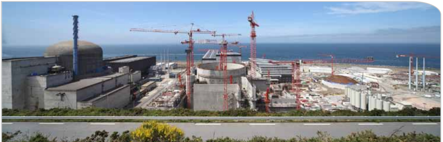
Flammanville 3 construction site - September 2011 - ©EDF
