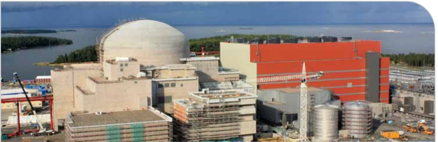
General view of Olkiluoto 3 construction site, Finland - September 2011
