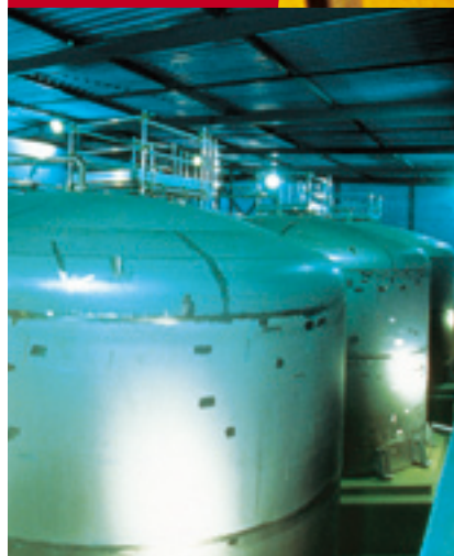
REPROCESSING NUCLEAR FUEL T3 AND T5 FACILITIES
