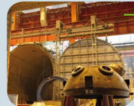
Heat treatment of a steam generator channel head
